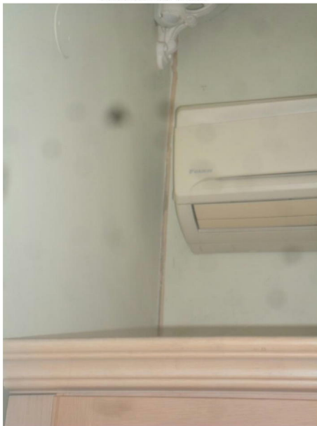
Subsidence crack
