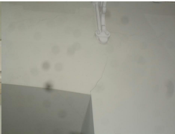
Subsidence crack
