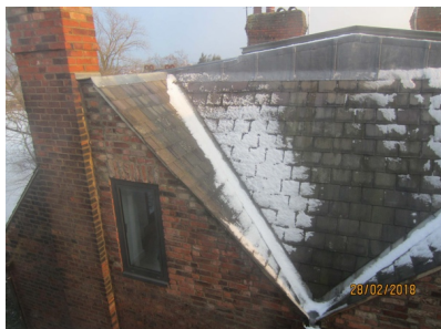
15 Tanza Road taken from communal stair window at 17 Tanza Road
