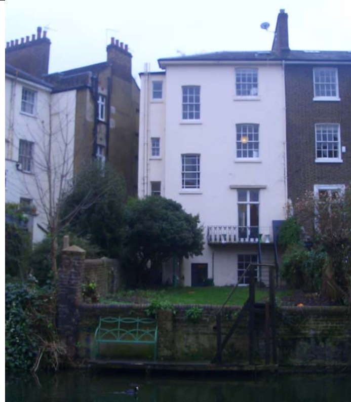
Figure 1: Rear View of property
