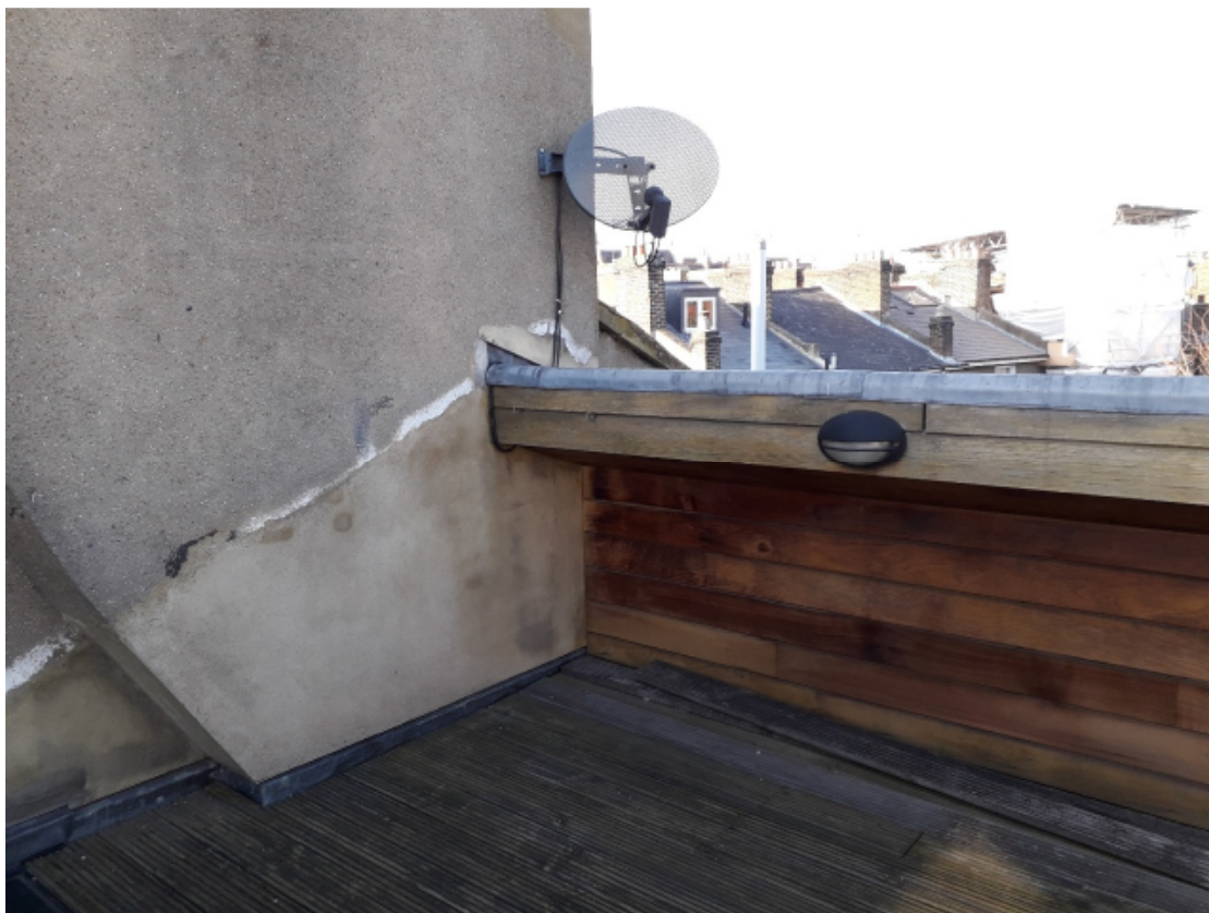
3. Roof terrace view facing rear elevation
