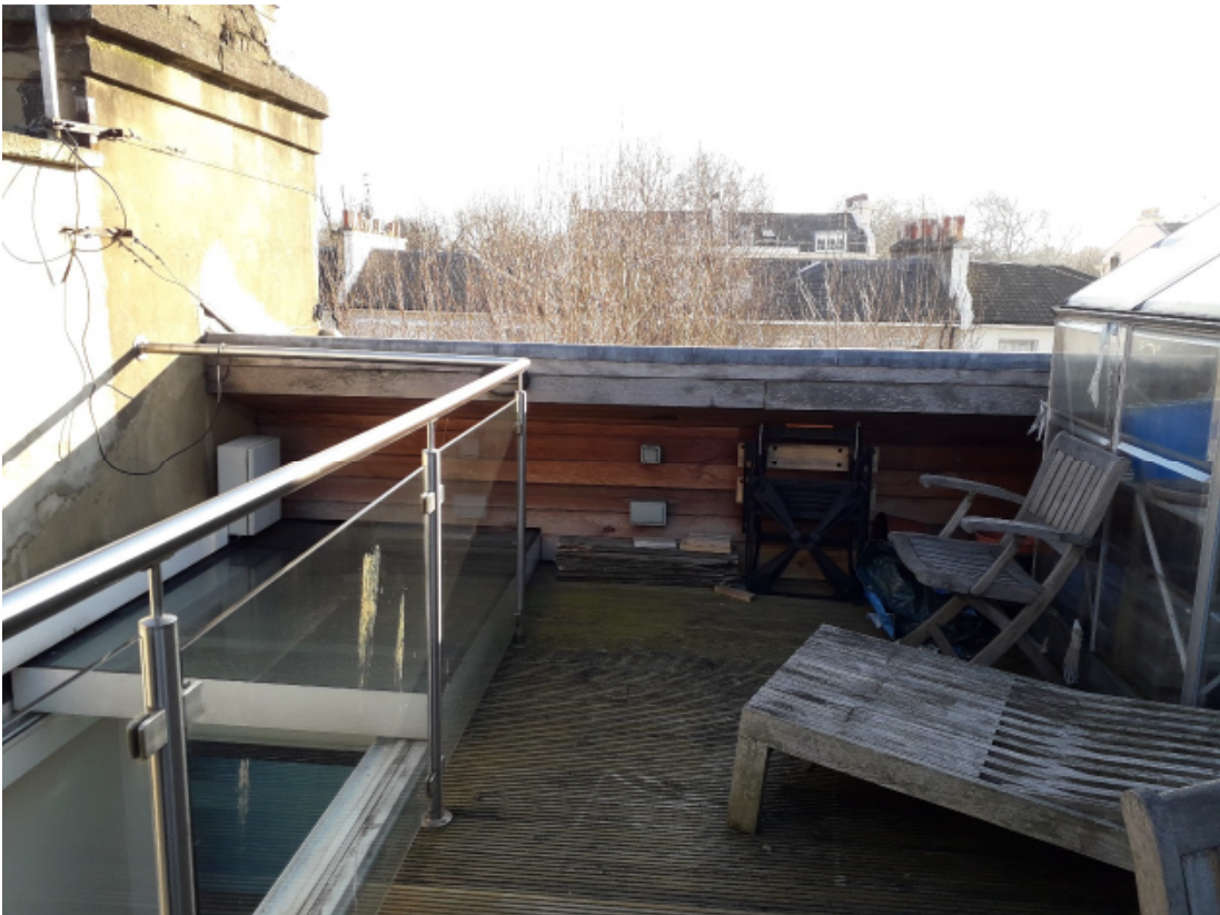
2. Roof terrace view facing front elevation
