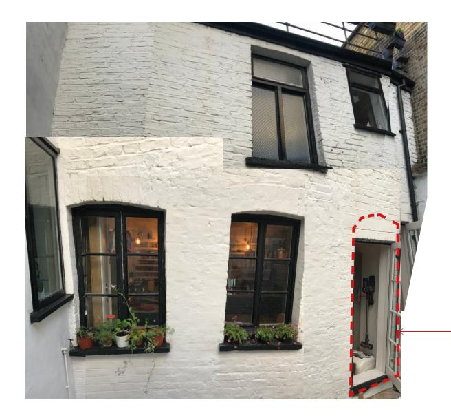
Area in dotted line is the only new brickwork.
