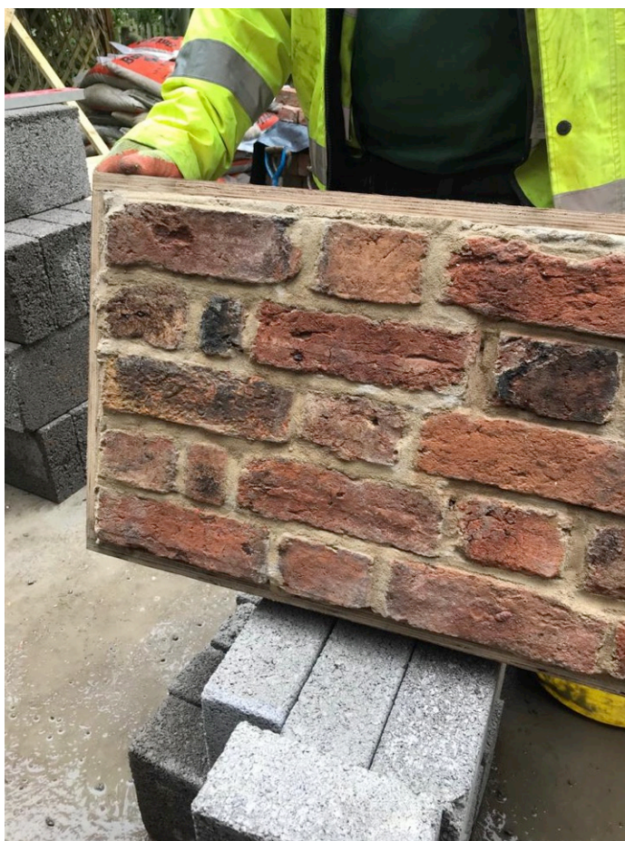
Sample panel of Brickwork, re-using original bricks with lime mortar and flush pointing
