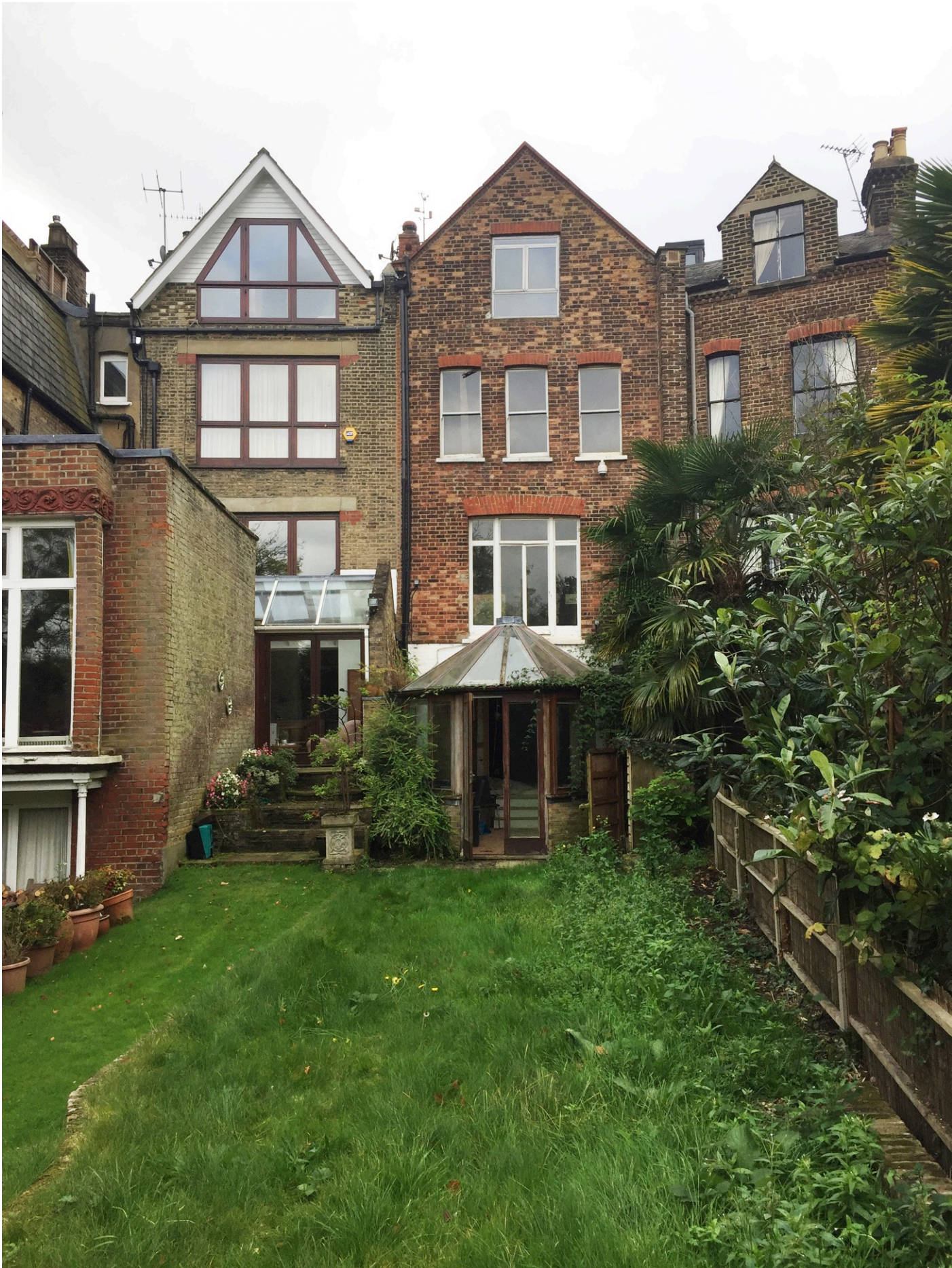
Rear elevation of Hillview prior to works commencing
