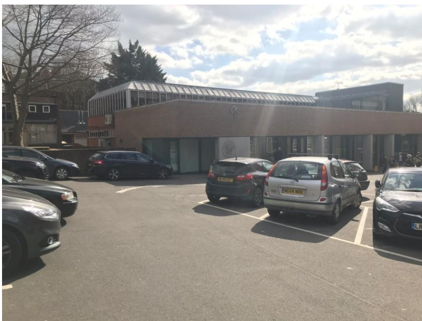
Fig.6 Sixth Form Centre as seen from north-east within parking area
