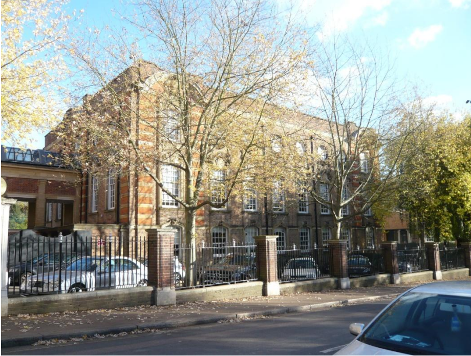
Fig.3 South Block as currently seen from road (west facade)
