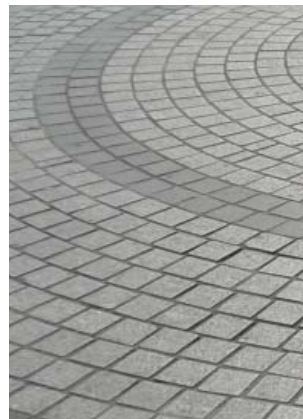
Fine picked silver grey granite sets in stretcher bond
