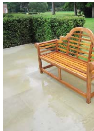
York stone paving to match existing
