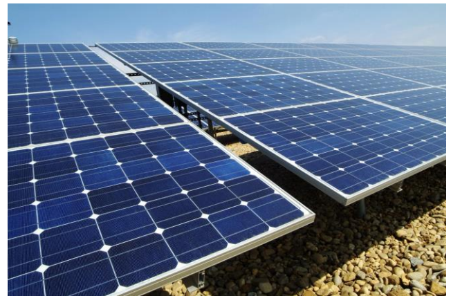
Figure 5: Monocrystalline PV arrays
