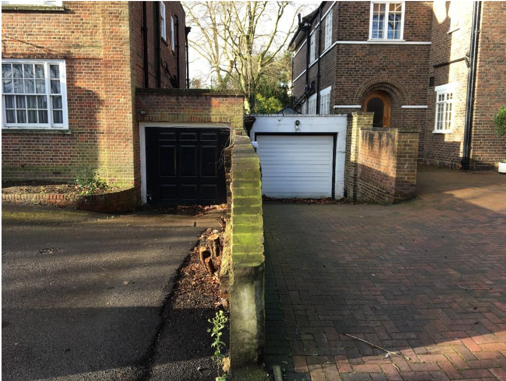
Main property and garage level differences at No. 73-75 (left) and No. 77 (right)
