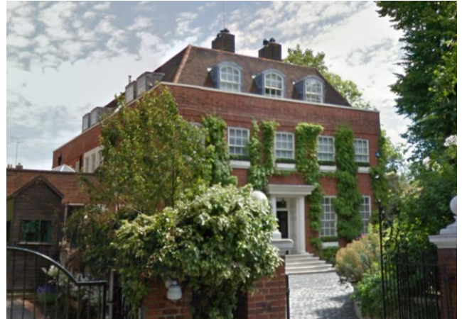
Figure 10: 56 Avenue Road Windows
