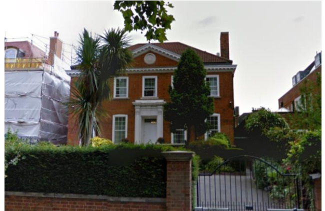
Figure 8: 58 Avenue Road Windows
