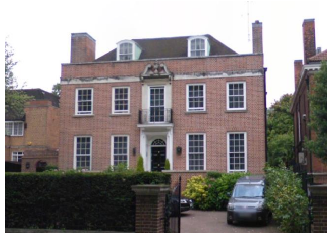
Figure 6: 60 Avenue Road Windows
