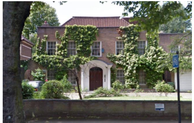
Figure 2: 79 Avenue Road windows
