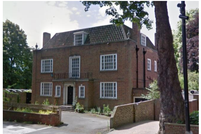
Figure 4: 75 Avenue Road Windows
