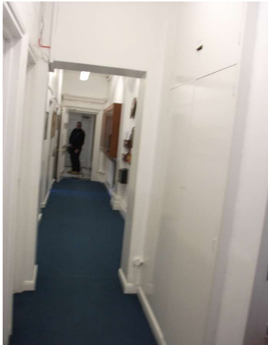
Photograph showing a corridor in the Centenary Building; The layout is a warren of tight corridors with little natural daylight.
