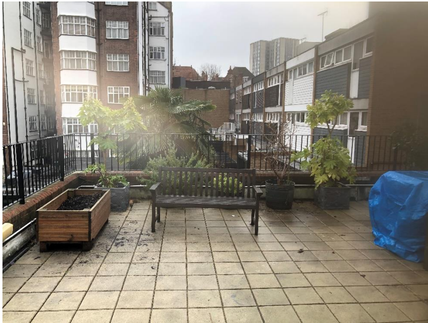
Photo 1. Patio section joining Building 1c and 1d with introduced shrub planters visible.
