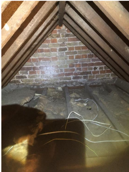
Photo 5. First loft void within Building 1a
