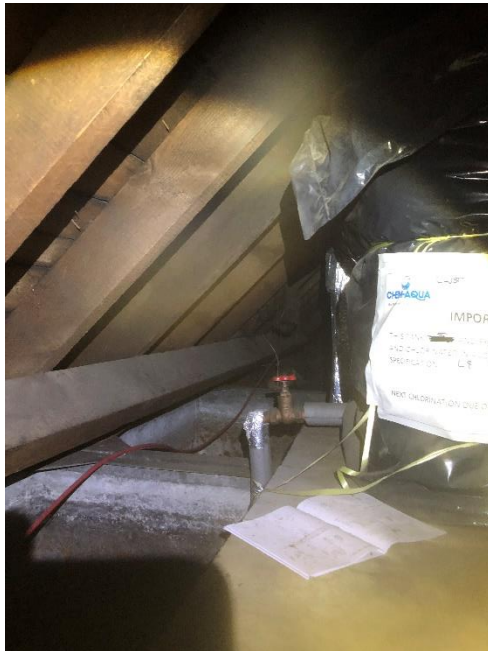
Photo 6. Second loft void within Building 1a
