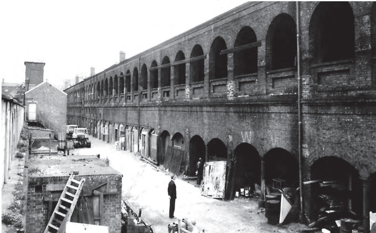
Figure 8 (opposite): The St Pancras area in about 1820 showing the Regent's Canal and open fields where Coal Drops Yard now stands Figure 9 (above): View of the eastern elevation in about 1980
