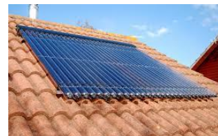
Figure 6 – Solar Thermal Panels
