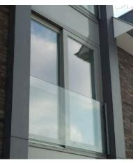
5- CLEAR GLASS BALUSTRADING, ALUMINIUM PANELS & SLIDING DOORS TO FRONT ELEVATION (or similar)
