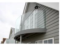
4- 1.8M HIGH FROSTED CURVED BALUSTRADE TO REAR ELEVATION (or similar) Type: frosted toughened glass Size: 1.8m high
