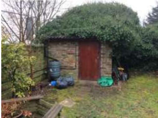
Image 5: Brick built shed with metal roof
