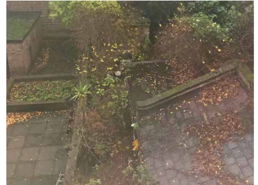
VIEW OF GARDEN FROM SECOND FLOOR
