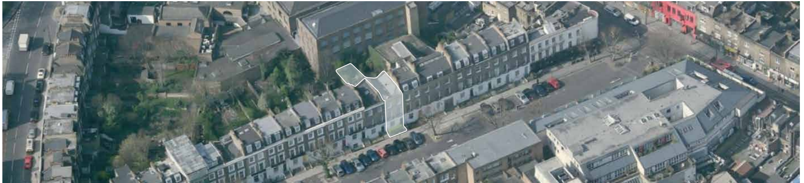
AERIAL LOOKING WEST
