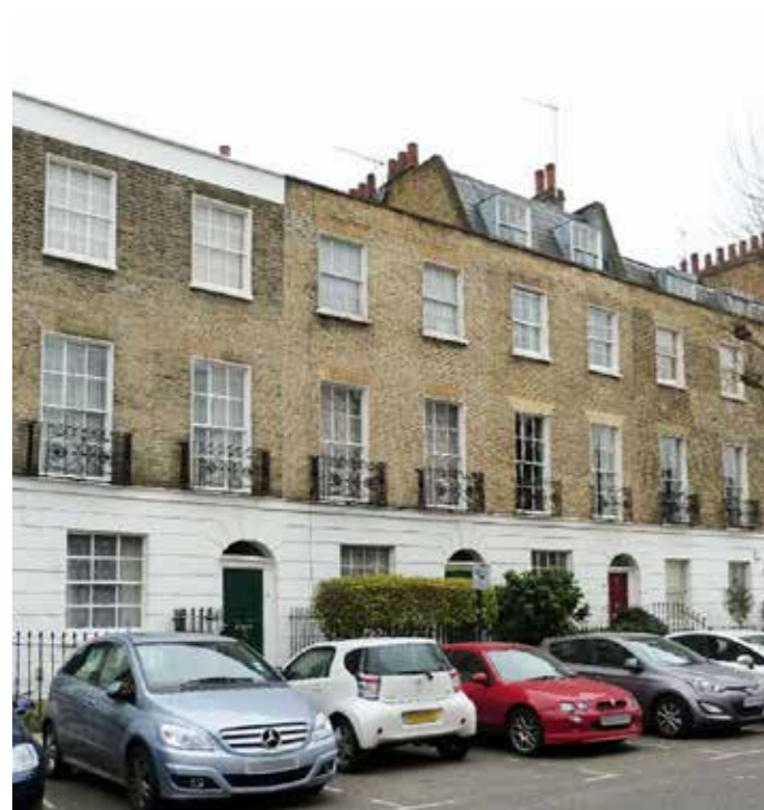
EXISTING BUILDING, FRONT VIEW
