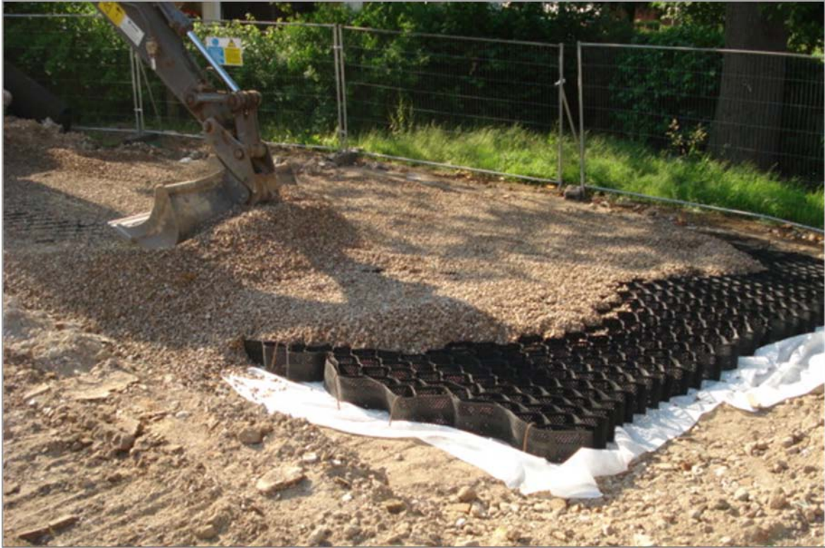
Figure 1. – Photographs of reduced-dig 3D webbing and ‘ArborRaft’ crate system ground protection.
