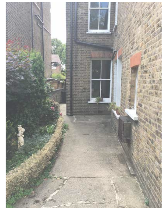
existing side entrance
