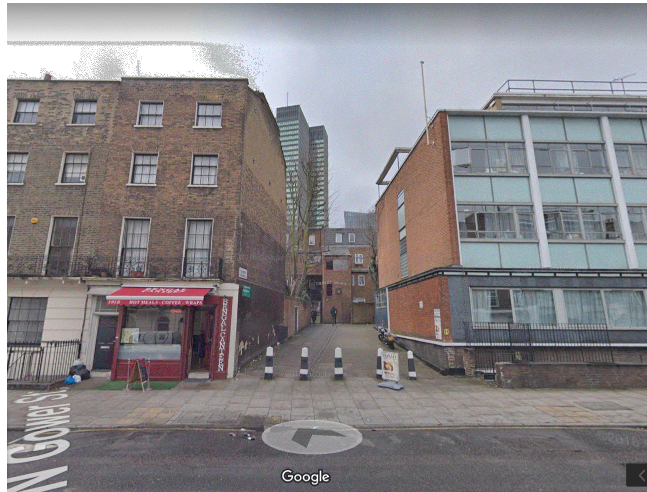
Gateway - B. View from North Gower Street showing pedestrian access.
