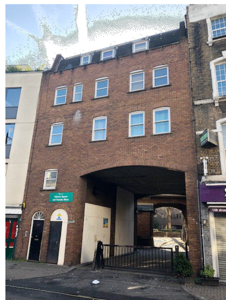
Gateway - C. View from Drummond Street showing vehicular & pedestrian access.
