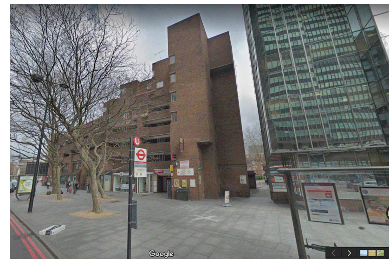
Gateway - D. View from Hampstead Road showing pedestrian access.
