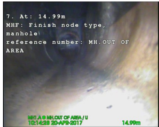
, 00:01:26, 14.99m Finish node type, manhole reference number: MH.OUT OF AREA
