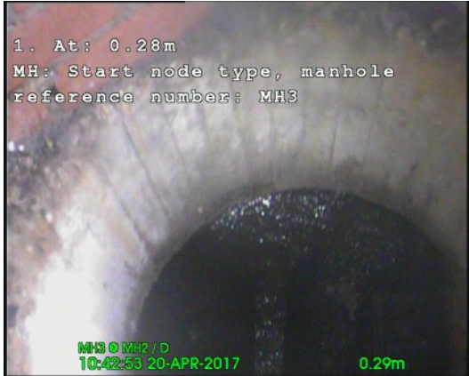
, 00:00:05, 0.27m Start node type, manhole reference number: MH3
