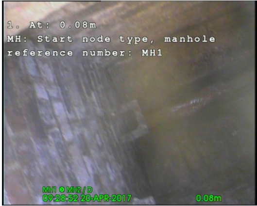
, 00:00:12, 0.08m Start node type, manhole reference number: MH1
