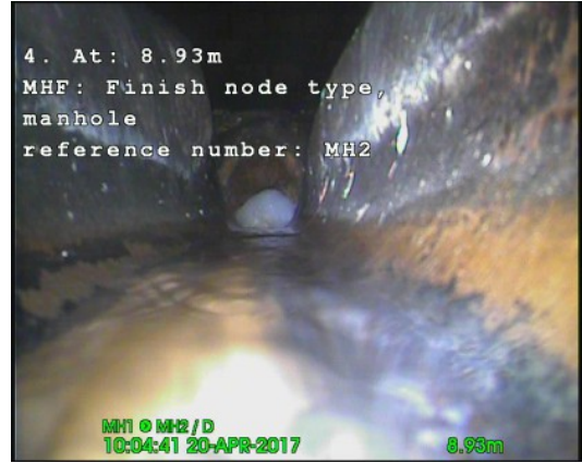
, 00:02:38, 8.93m Finish node type, manhole reference number: MH2
