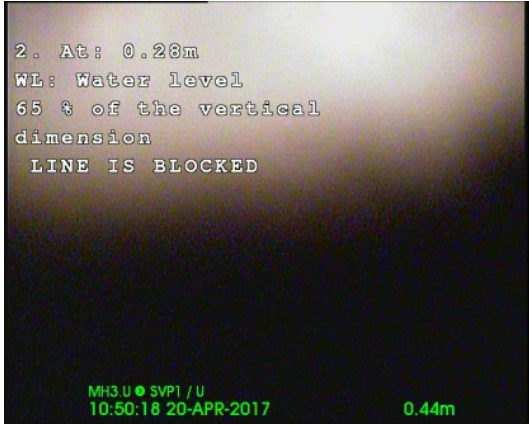
, 00:00:03, 0.44m Water level 65 % of the vertical dimension LINE IS BLOCKED
