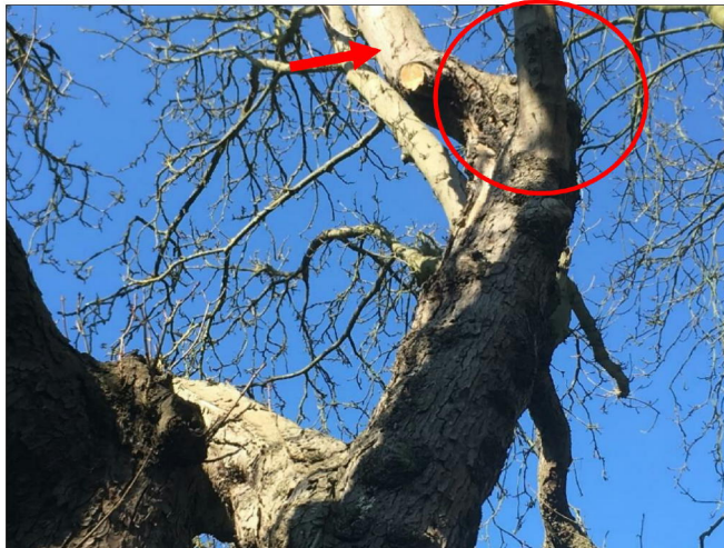
Fig. 4 Circled – a weak and decayed union between the relatively new stem/spar (arrowed) and the parent stem/trunk
