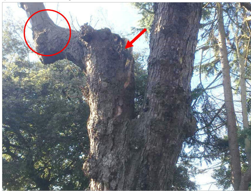
Fig. 5 Extensive decay has developed at an historic pollarding location (arrowed); circled weak spar/stem union under high stress.
