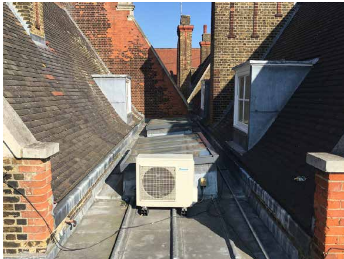
Fig 4.5.1. A new condenser and ventilation cowls will be located between the two rooflights.
