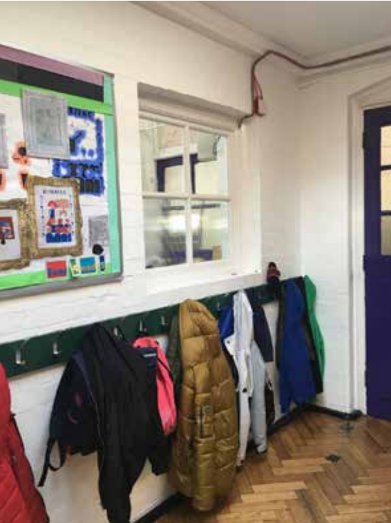
Fig 4.4.7. The window to be lowered to form access to the Sensory and Soft Play Rooms.
