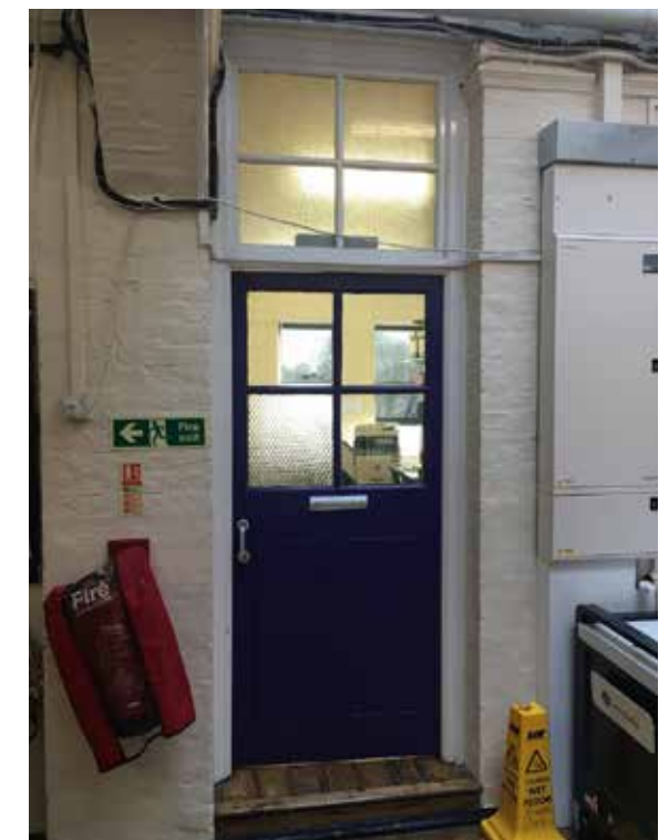
Fig 4.4.13. The door to the new WCs to be removed for re-use elsewhere. The frame and glazed panel over will be retained.
