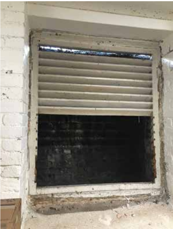
Fig 4.1.4. The damaged louvred opening.
