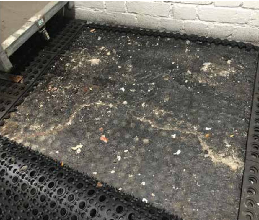
Fig 4.1.7. An area of floor with cement slurry and bituminous coating.
