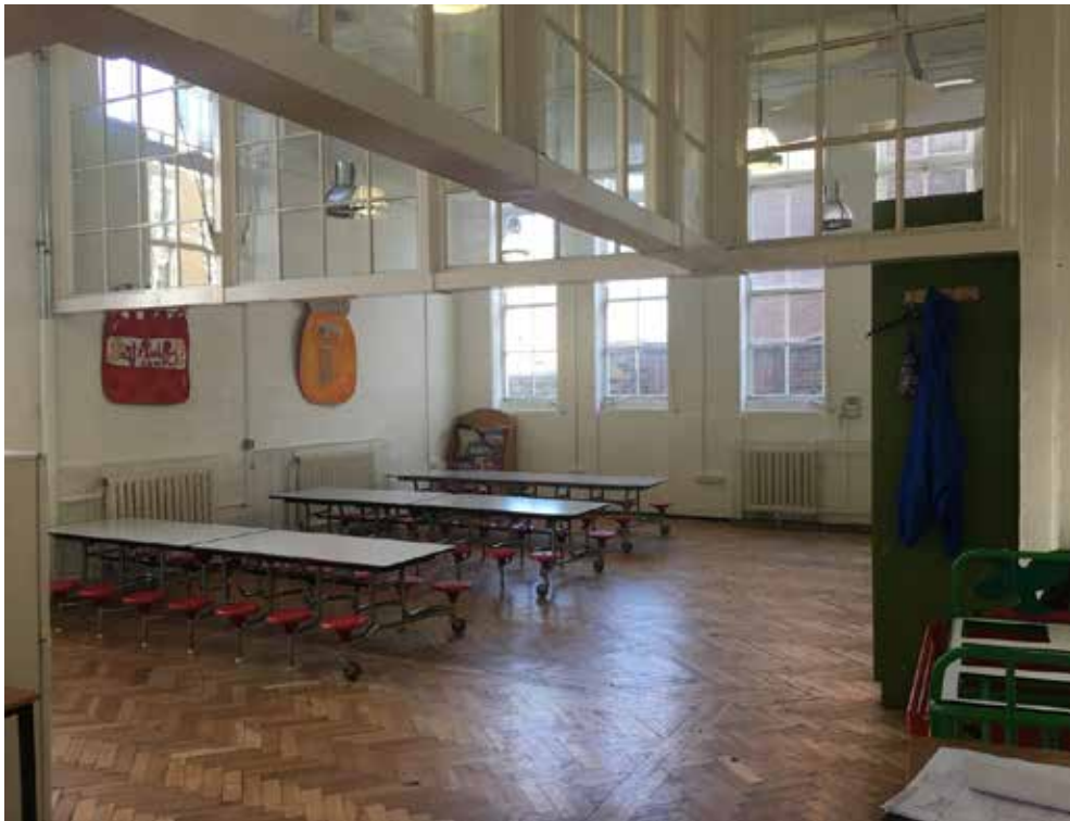
Fig 4.2.5. The ground floor dining area with 'floating' steel frame that supports original glass screens over..
