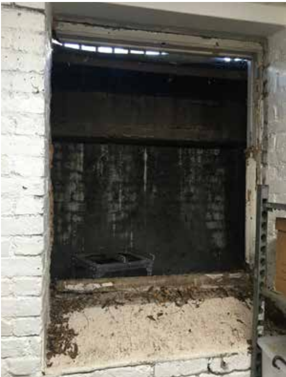
Fig 4.1.3. The damaged sash window. The glazed brick retaining wall is to be cleaned.
