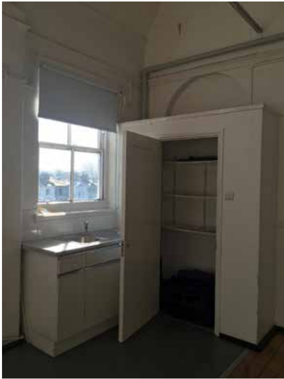
Fig 4.4.6. Kitchenette and cupboard in Rooms 44.0 and 42.7 to be removed. The cupboard has been reclad with plasterboard. The skirting will be realigned continuously along the wall.
