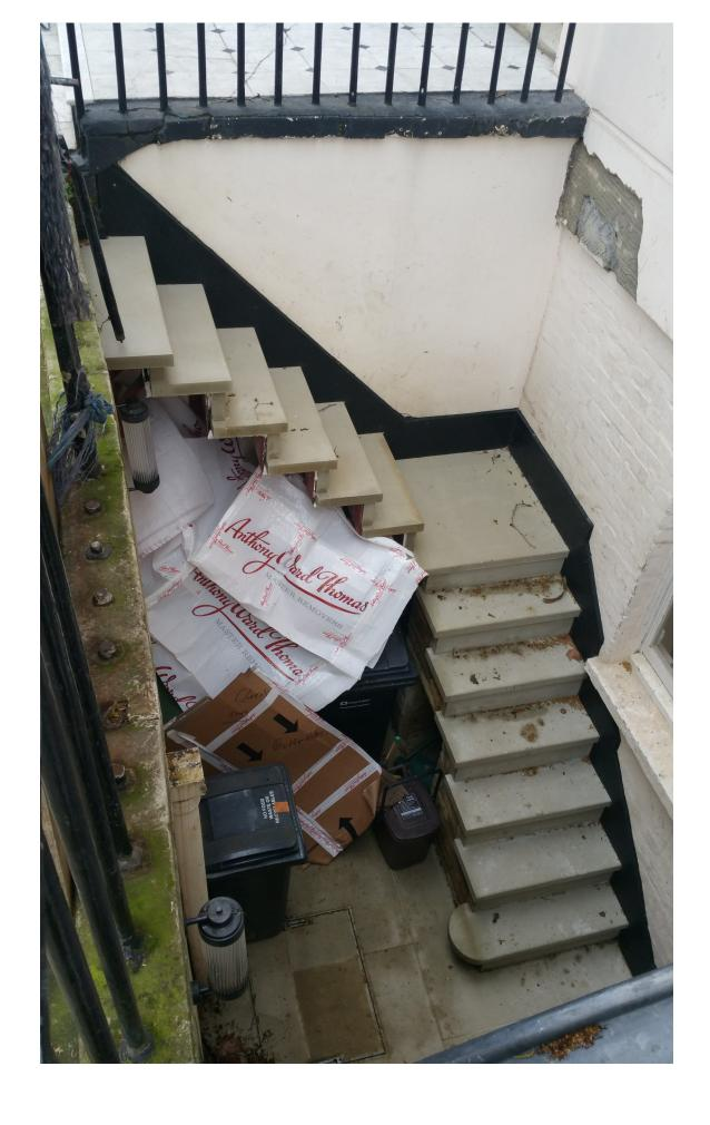
AREA STAIR REPLACEMENT UNDER CONSTRUCTION WITH YORK STONE TREADS RISERS AND LANDING February 2019
