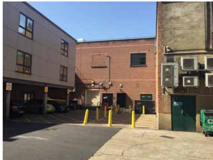
Rear elevation of building from the courtyard
