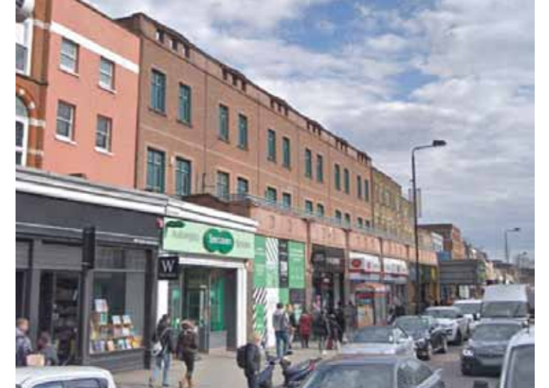
Main elevation as seen from the North on Camden High Street
