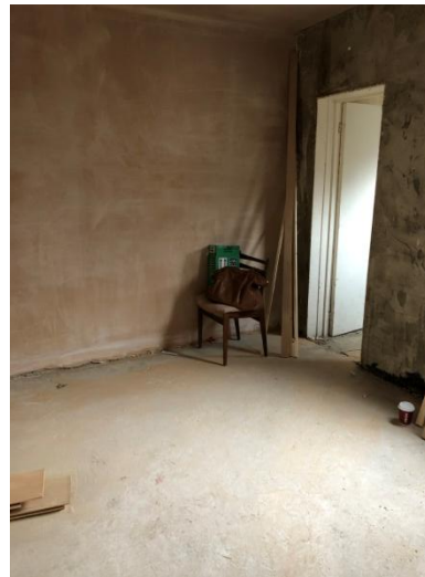
New concrete floor
