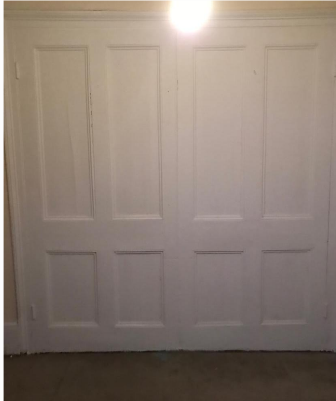
Fig 28 The original four panelled doors that were installed within the spine wall at 1 st floor level.
