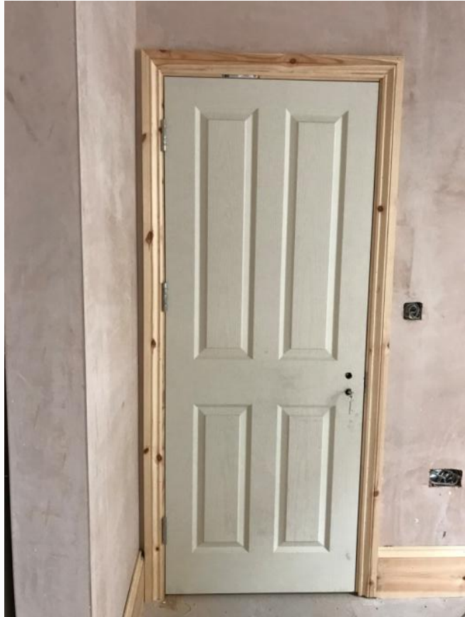
Fig 42 The inserted four panelled doors and new architrave.
