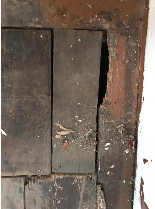
Fig 30 Badly damaged floorboards and evidence of decay from woodworm.
