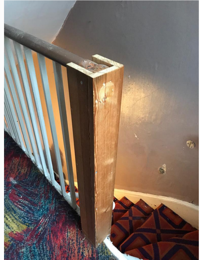
Fig 23 The newel post and balusters at 1 st floor landing level.
