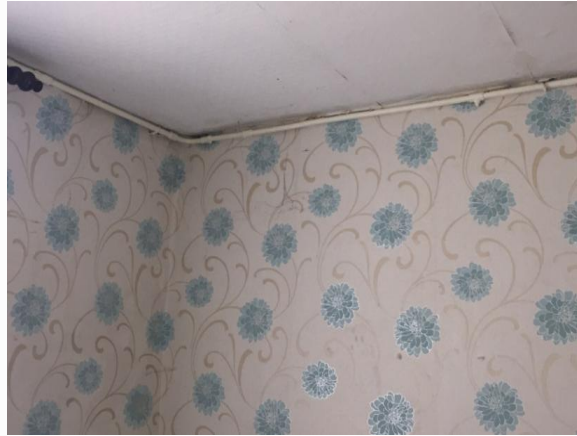
Fig 32 Surface mounted piping at high level to the ground floor rear room.
