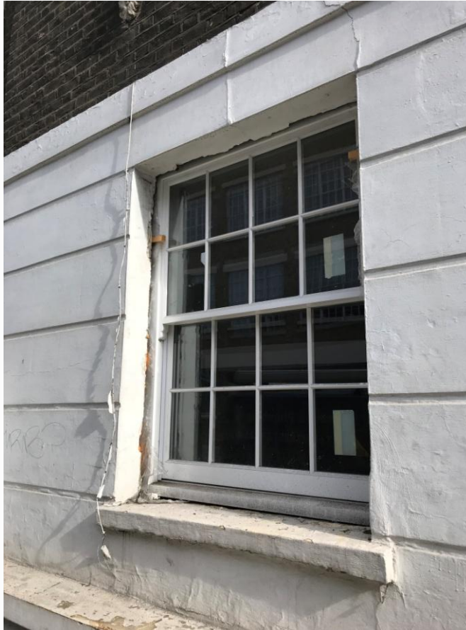
Fig 40 The newly inserted timber sash window to the front ground floor room.
