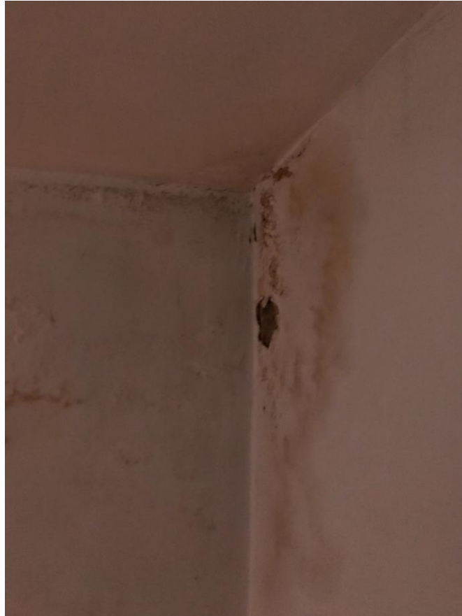
Fig 16 Significant damage to plaster finishes due to water penetration.
