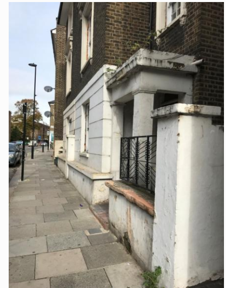
Fig 15 The lower part of the front facade showing deterioration of finishes.
