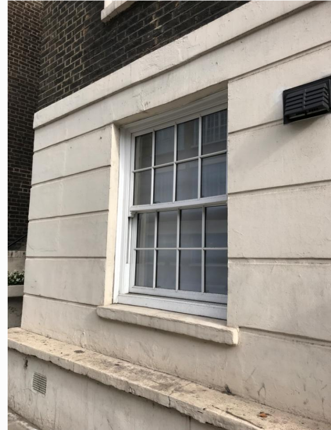
Fig 39 The PVCu double glazed window to the ground floor of no.70 Highgate Road.
