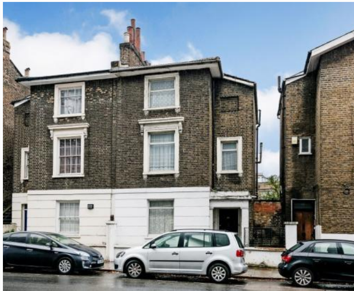
Figs 47 and 48. The modern section of brickwork shown above to the right of the property and the newly repaired area at Fig 48.
