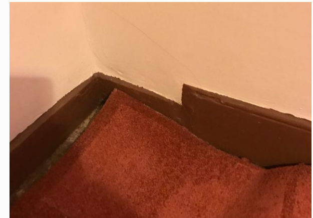
Figs 35, 36 and 37. Mismatched skirting of different heights and profiles, showing significant damage, wear and tear and distortion. Fig 35 shows where timber skirting had been replaced with painted cement.
