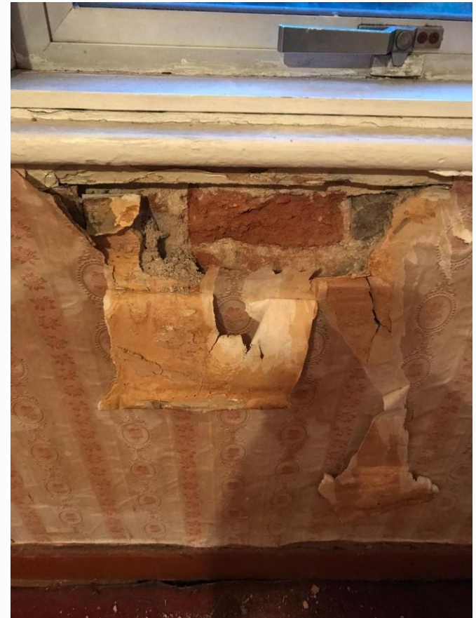
Fig 17 Damage to wall and plaster finishes at 2 nd floor level.
