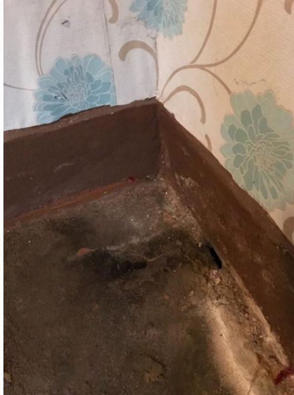
Figs 35, 36 and 37. Mismatched skirting of different heights and profiles, showing significant damage, wear and tear and distortion. Fig 35 shows where timber skirting had been replaced with painted cement.
