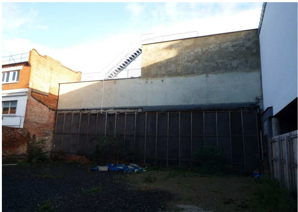
Figure 4: View northeast at boundary wall with 246 Kilburn High Road
