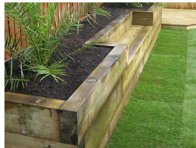
05 | Oak sleeper retaining wall
