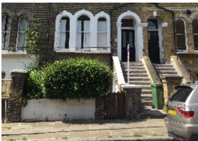
Dilapidated wall with wooden gated access to 23A. Unsightly asphalt finish to steps. No bin storage.
