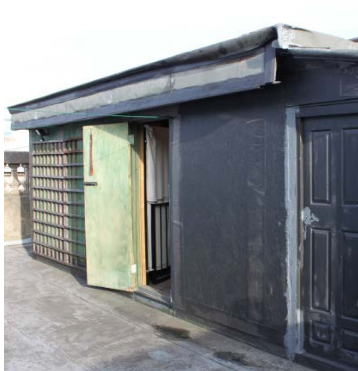
1. Access onto roof from fourth floor
