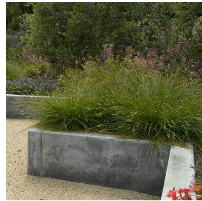
Concrete planter upstand
