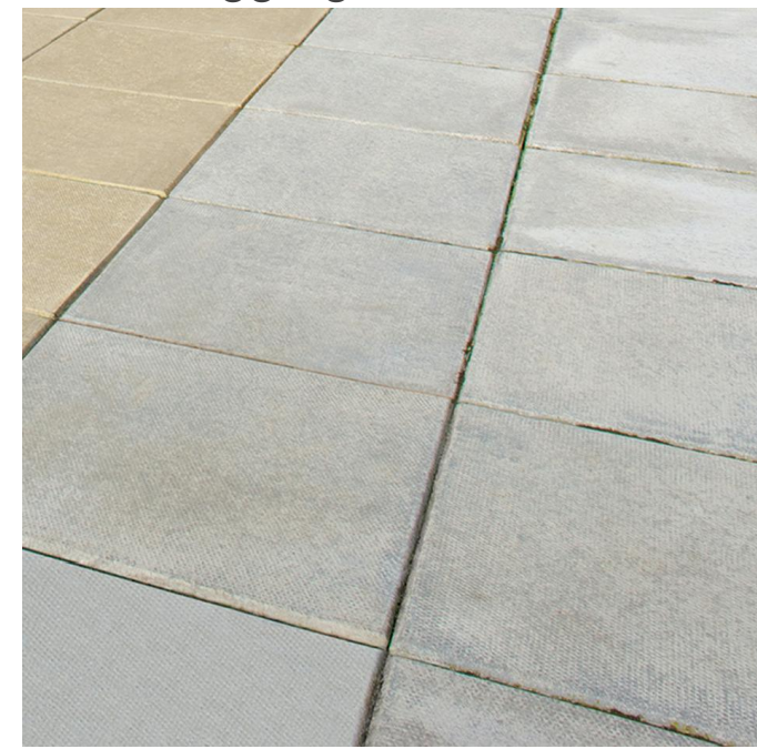
600mm BS PC Concrete paving.
