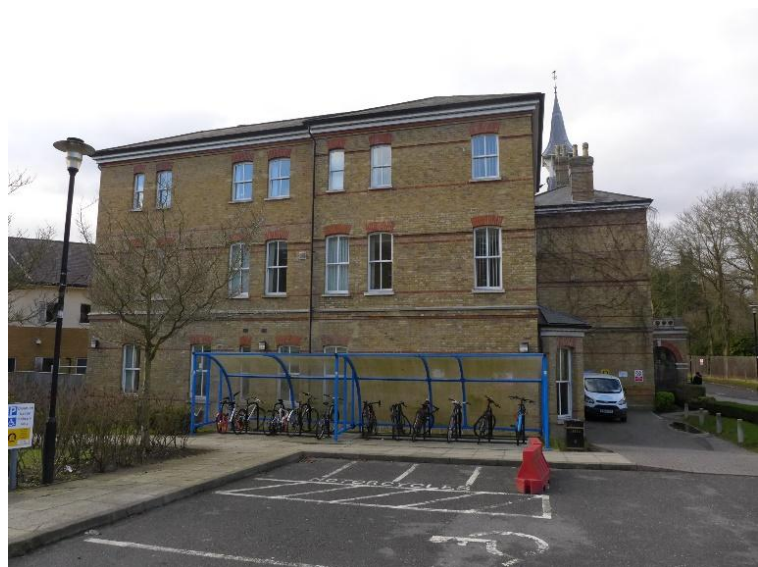
End elevation of Administration and Main Entrance block looking West
