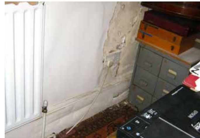
Image 4: Example of internal water ingress showing defective plaster and dry rot to skirtings
