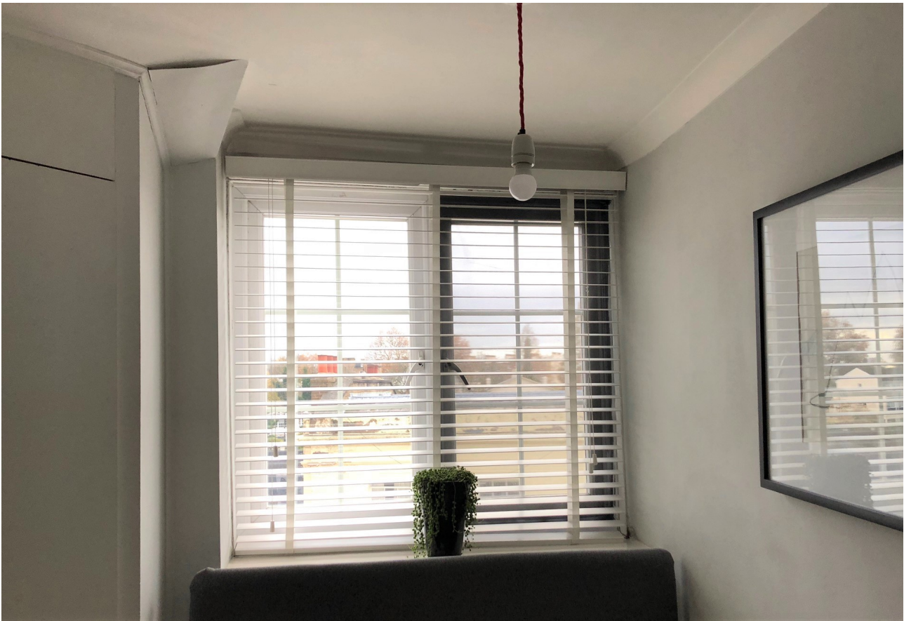
Figure 5: Internal view of window at third floor bedroom (Flat D)
