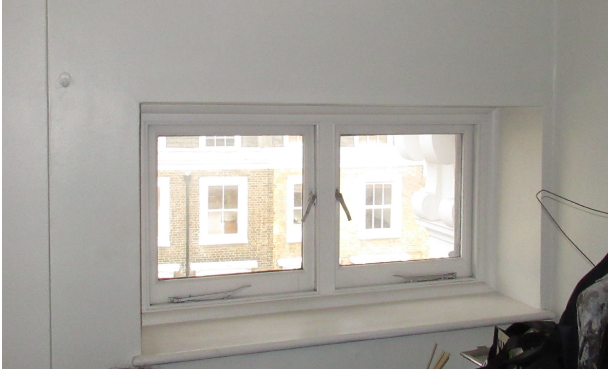
Figure 2: Internal view of window at third floor study room (Flat D)
