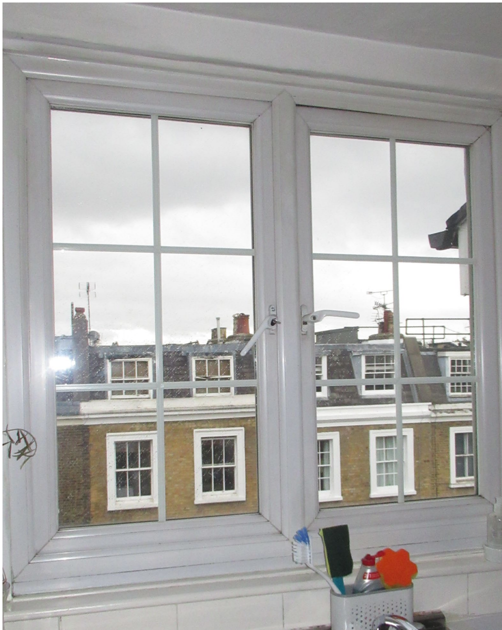
Figure 1: Internal view of window at third floor kitchen (Flat D)
