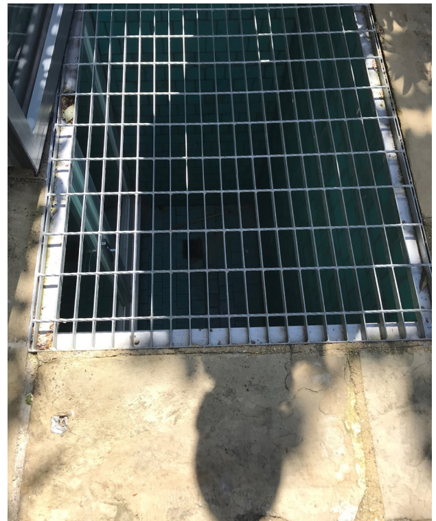
Lightwell grille cover directly outside main access to garden
