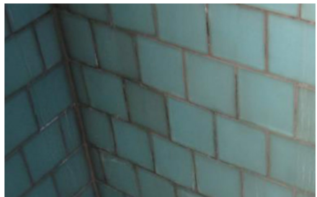
Top: Weak waterproofing point around metal grille over rear lightwell Bottom: Bulging wall tiles in the lightwell from water pressure buildup beneath the garden
