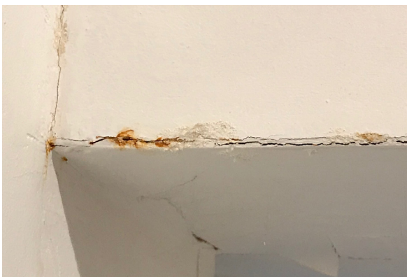
Top & bottom: water ingress into the room from above
