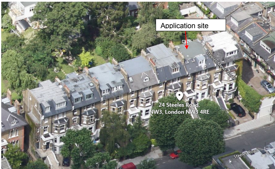
Photo 2: Ariel view of front of the application site and terrace of which it forms a part
