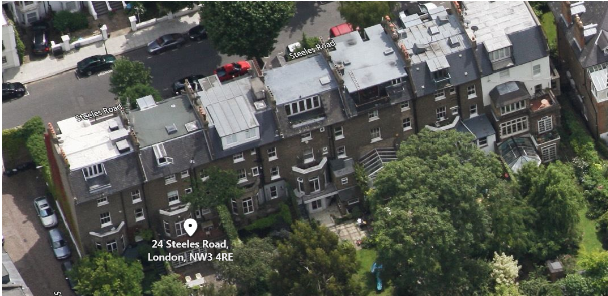
Photo 3: Ariel view of rear of the application site and terrace of which it forms a part
