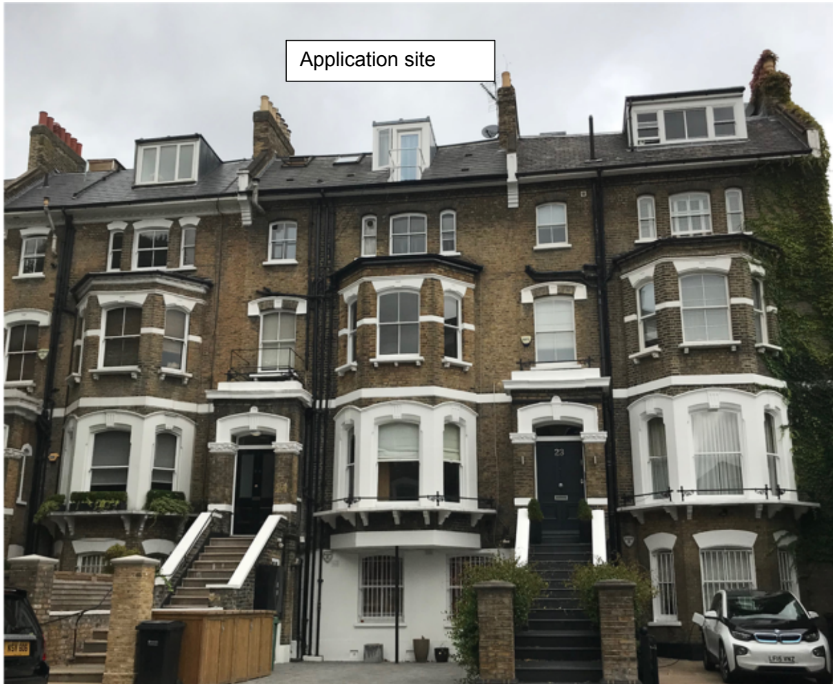
Photo 1: Front elevation of application site
