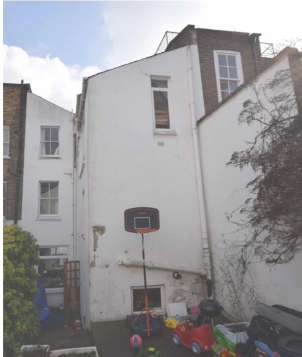
Fig 10: View of side elevation showing existing three storey extension interfacing with original outrigger and incongruous glazing
