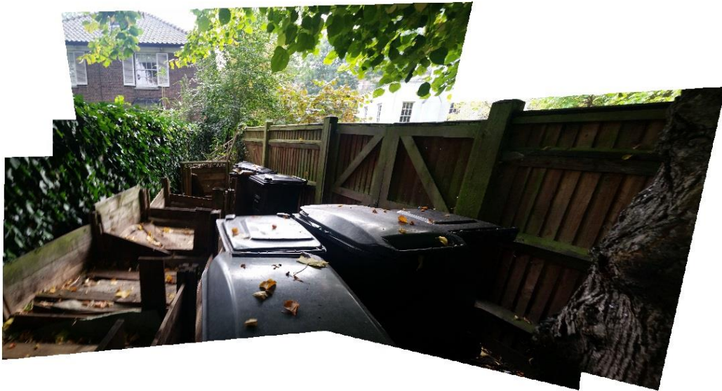
View of the existing bin store.
