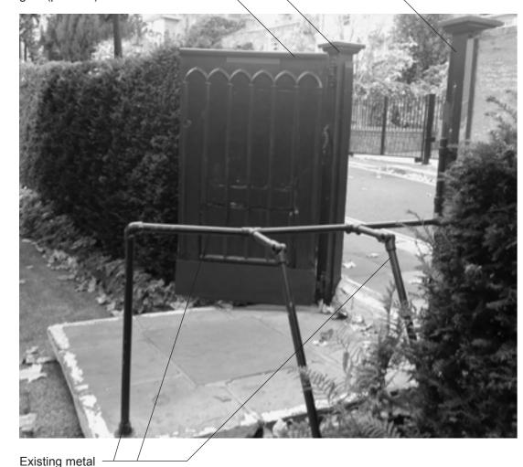
Recessed fixing into post to se details so fit for purpose without visible fixing plate Existing timber post retained Spigot welded into the handrail. Welds ground smooth to allow the hairline joint Flush screw on underside of the handrail Existing step with white line repainted with external 'grip' paint fit for purpose Base cemented into base and base chamfered up Base cast into R.C. base so all fit for purpose
