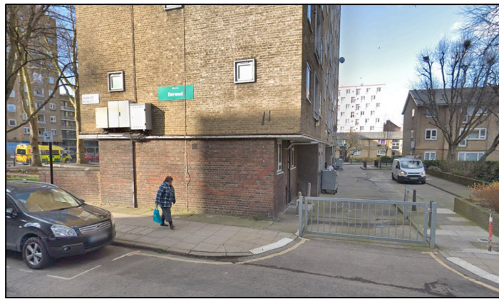
Existing wall Derwent
