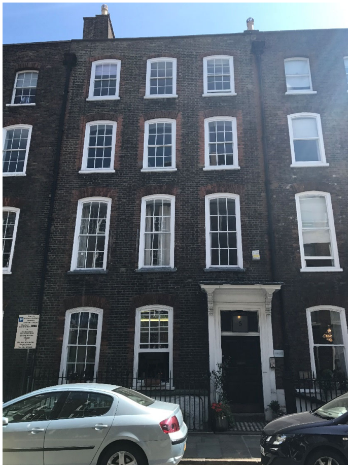
Fig 1 Street View: 5 Great James Street
