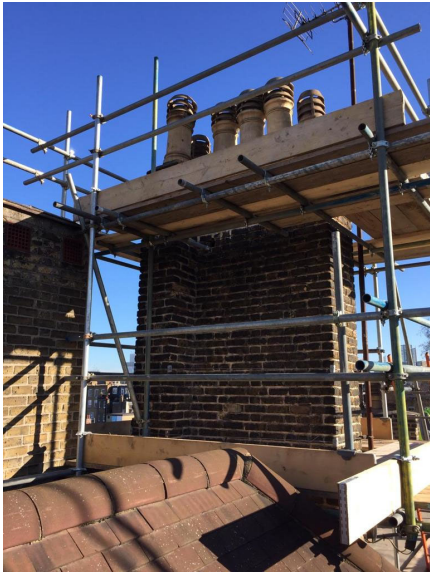
Fig 4 Chimney stack with supporting scaffold frame.
