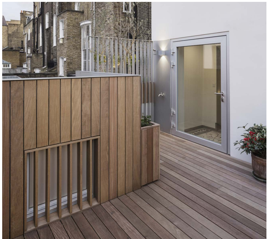
Ipe cladding/decking at 16 John Street, Bloomsbury by Prewett Bizley Architects
