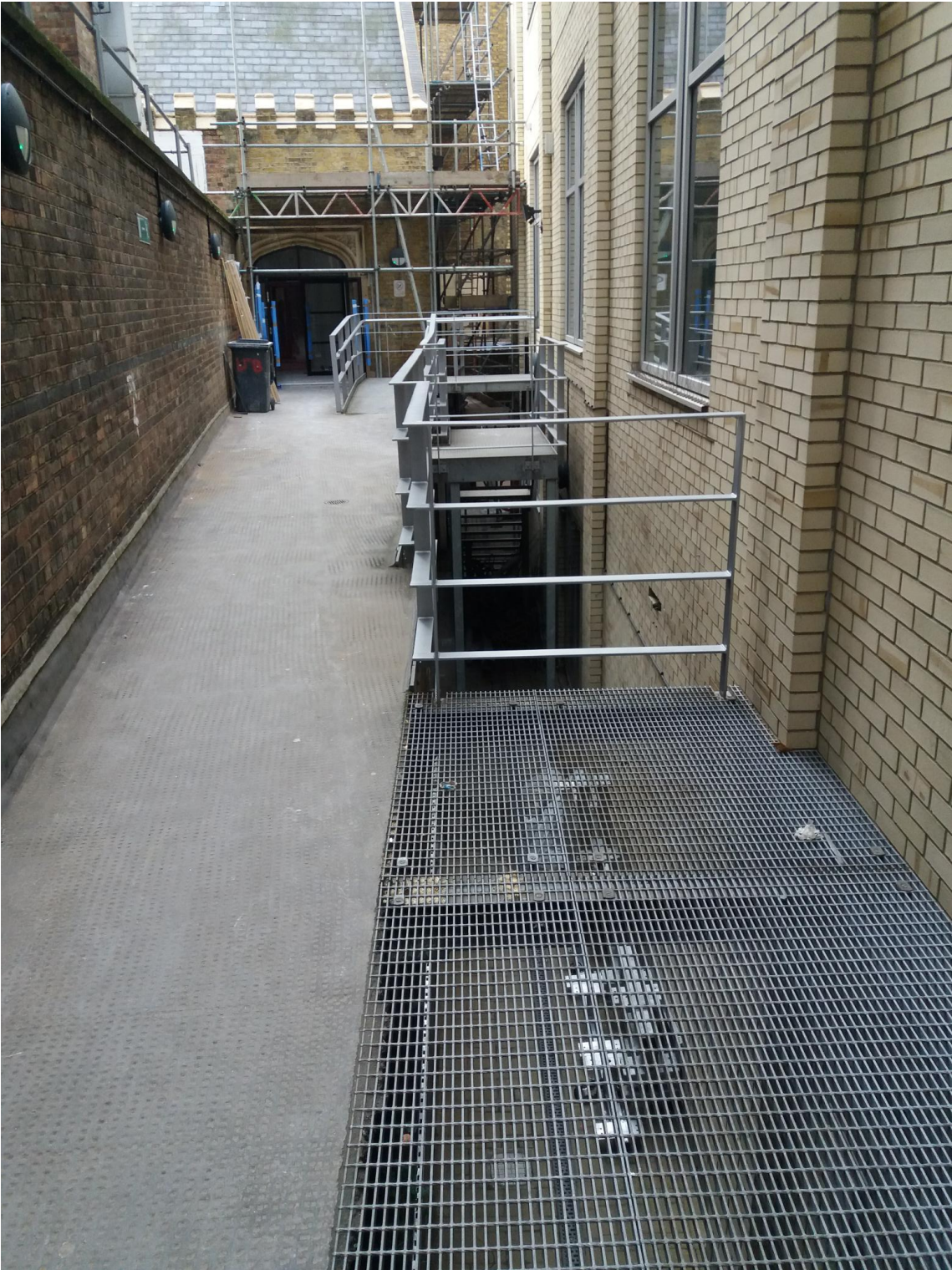
2. View of walkway and staircase towards chapel annex
