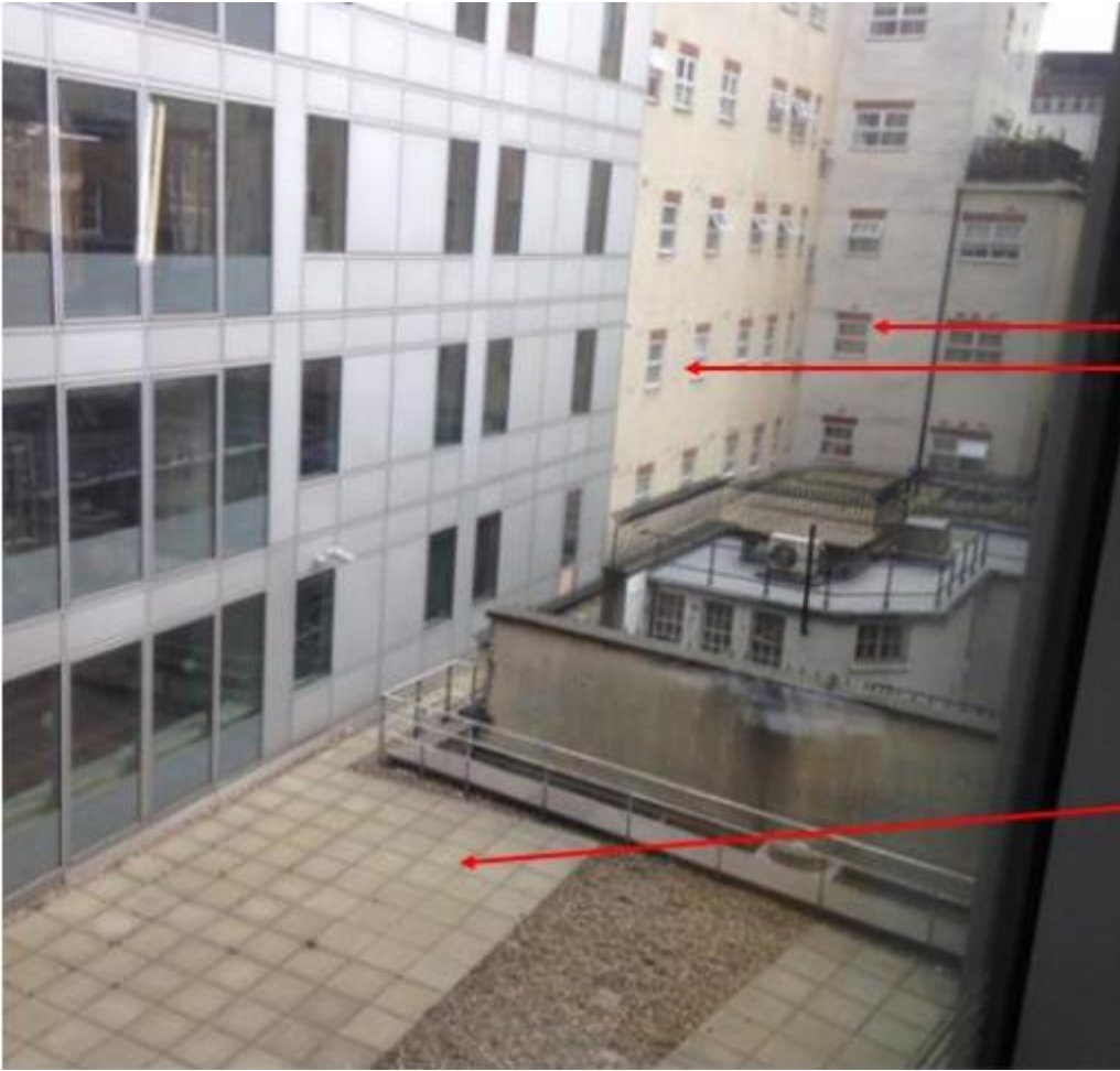
7. View from upper floor towards 1 st floor flat roof
