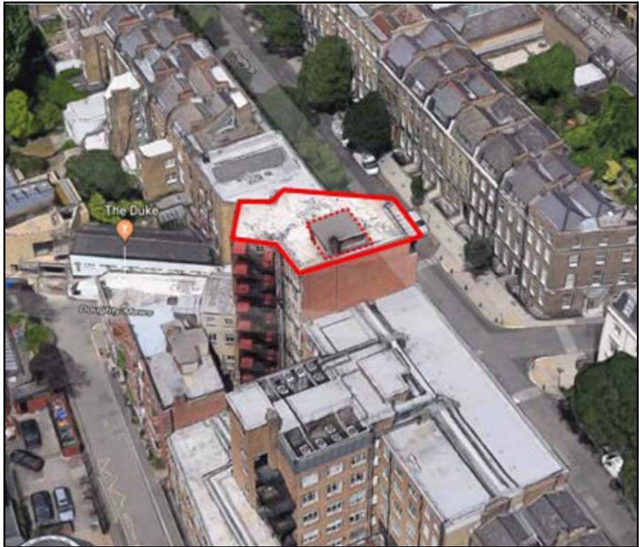
Red line outlines total area of the roof. Dotted line outlines extent of the current lift overrun.
