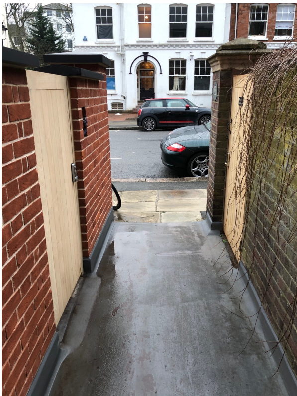
Photo showing gate to No. 23 (right) in context of neighbour gate to No. 23a
