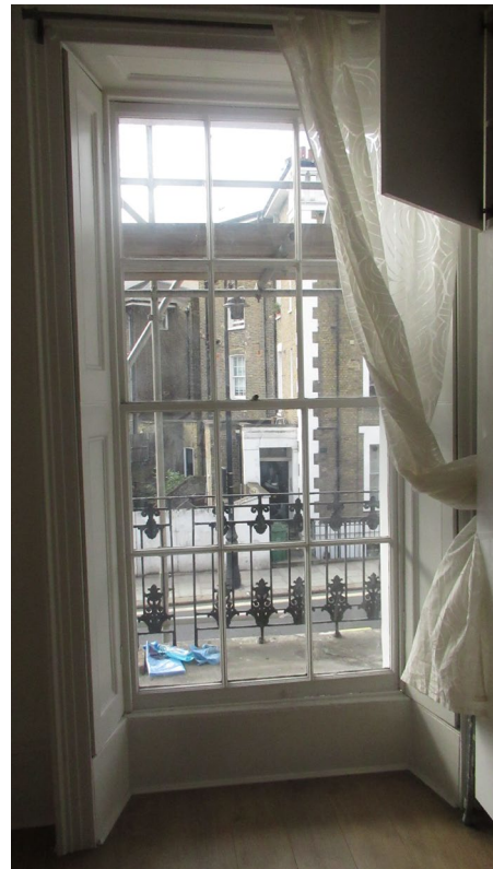
Figure 9: Internal window at first floor (R)
