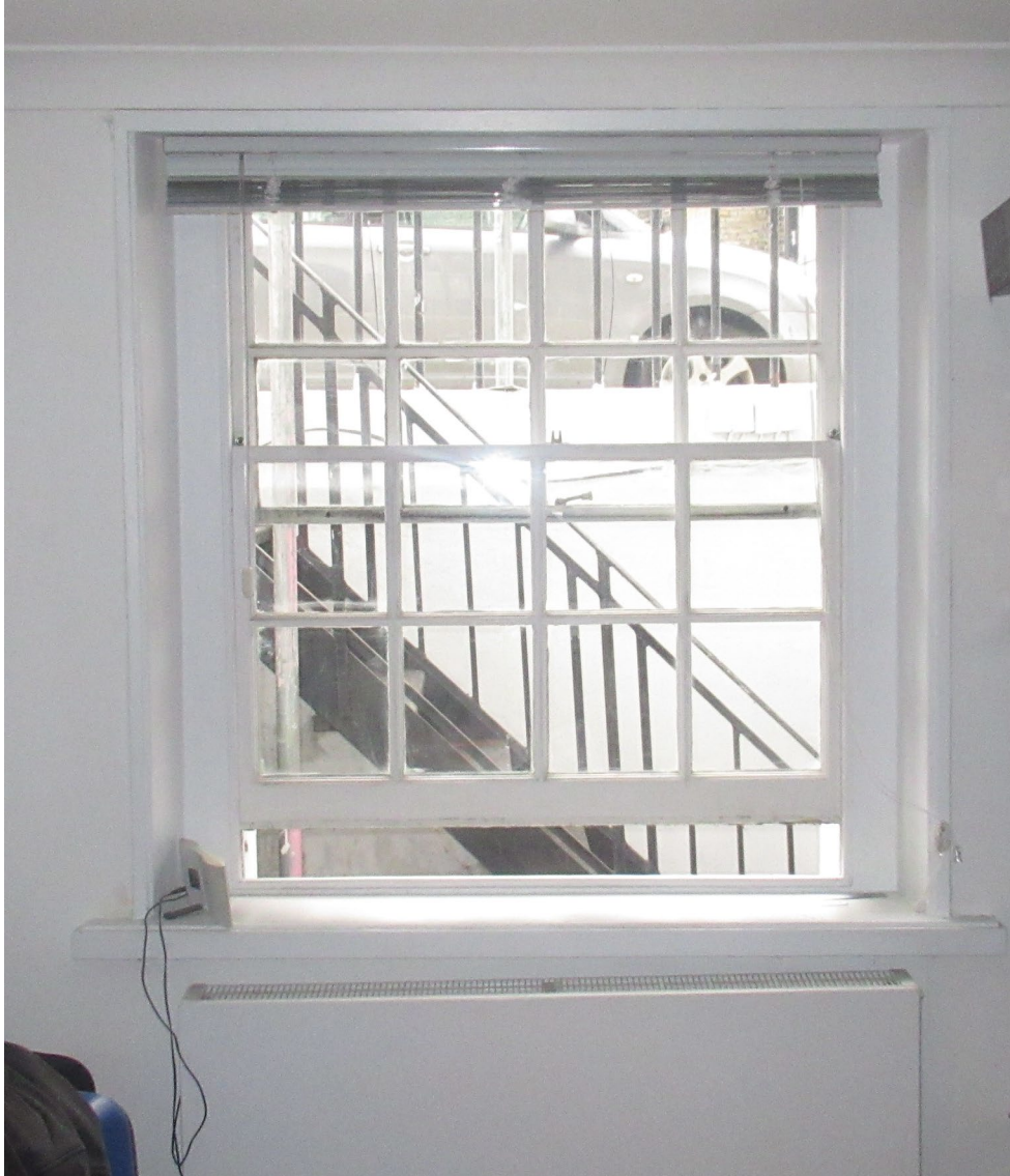
Figure 7: Internal view of the window in the bedroom at basement level
