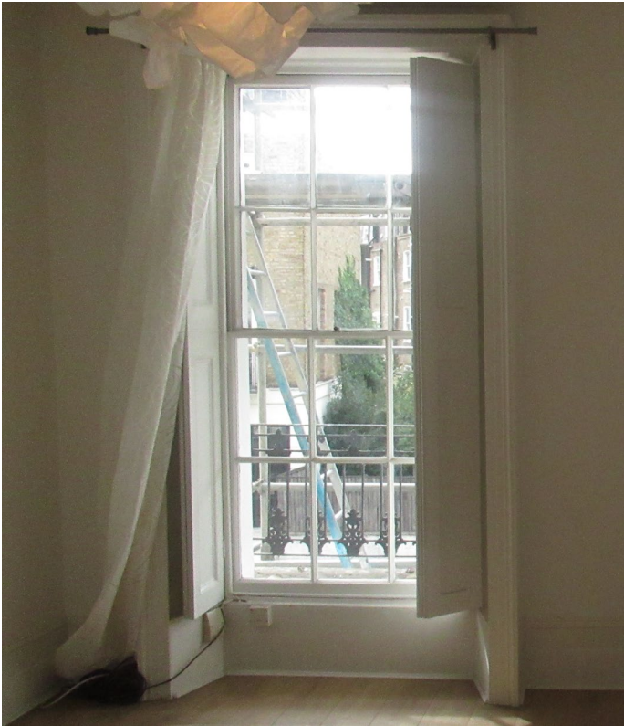
Figure 10: Internal window at first floor (L)
