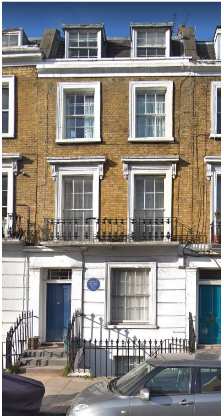
Figure 6: A view of south facing (principal) elevation of 54 Delancey Street
