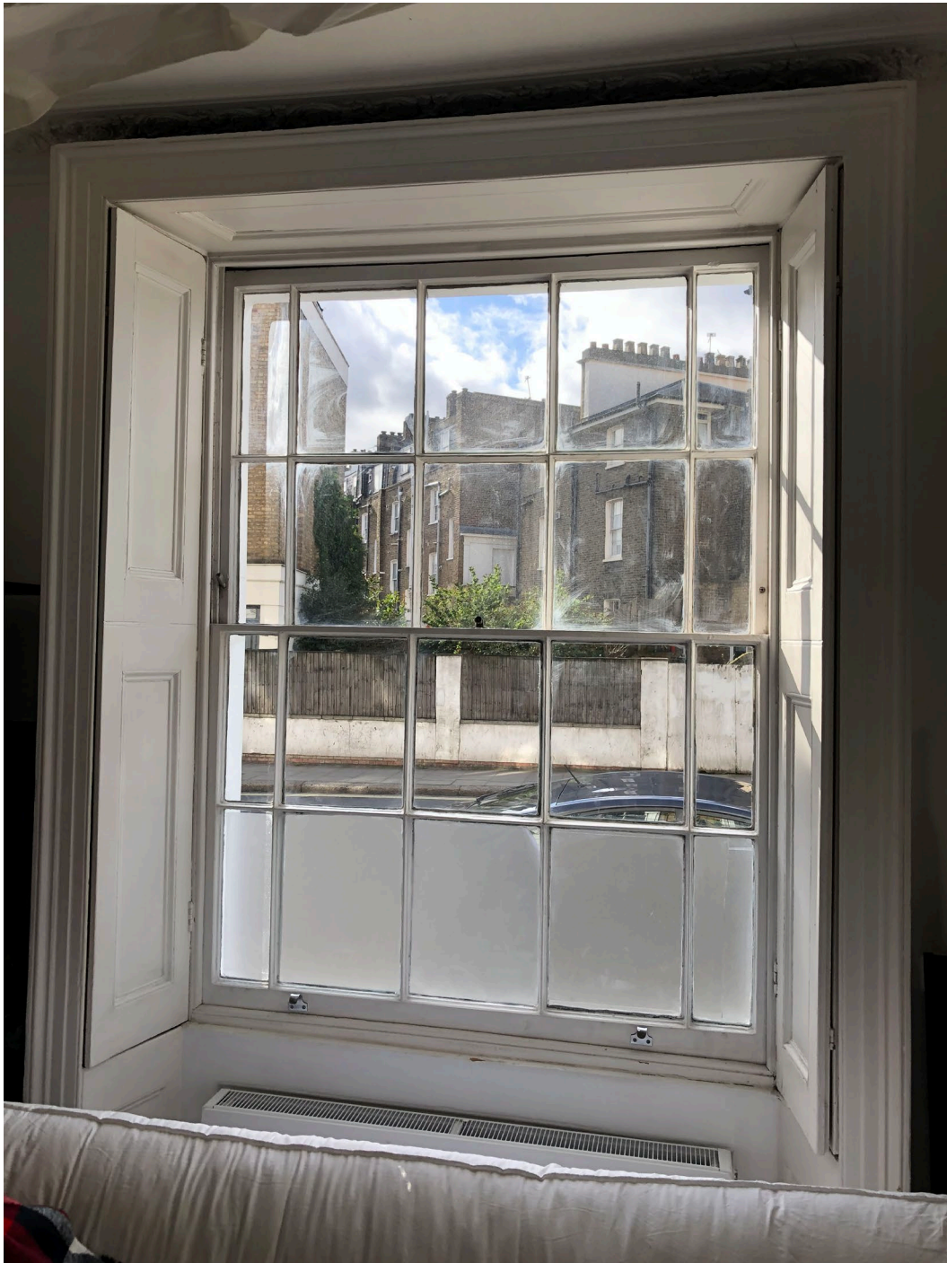
Figure 8: Internal view of the window in the ground floor living room
