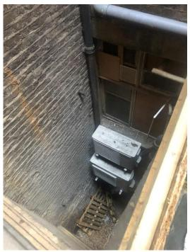
This application seeks to install replacement equipment at the site, specifically a new air handling unit and attenuation to the existing plant. Redundant plant will be removed. These alterations are proposed within an existing plant area in the rear lightwell. As such, the proposal will preserve the character and appearance of the conservation in accordance with Policies D1, D2 and Camden Planning Guidance 1: Design and not result in any harm to the significance of the listed building.
