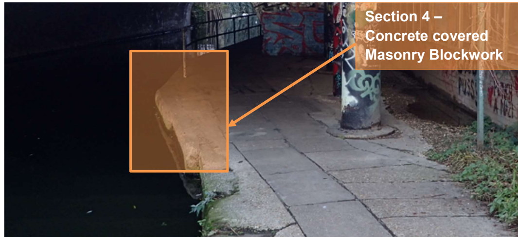
Figure 3.11: Photograph indicating Section 4 - Concrete covered Masonry Blockwork Wall
