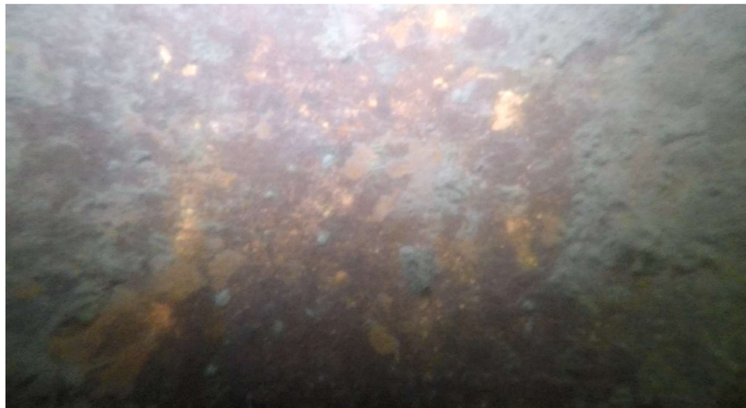
Figure 3.13: Photograph indicating a segment of the uncovered wall of Section 4
