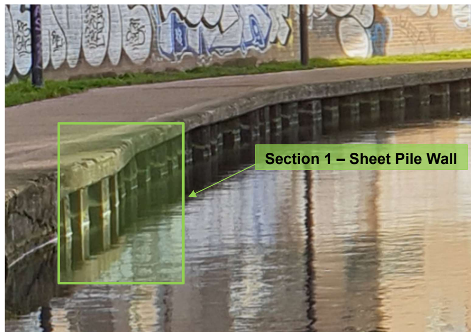
Figure 3.1: Photograph indicating Section 1- Sheet Pile Wall above water
